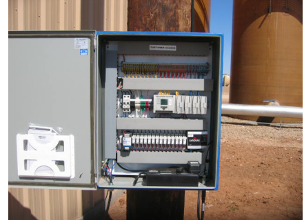
RTU consisting of MicroLogix 1100 PLCs, discrete I/O, and RadioLinx Industrial Hotspot
