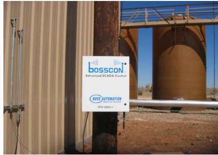
RTU consisting of MicroLogix 1100 PLCs, discrete I/O, and RadioLinx Industrial Hotspot
